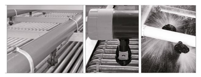
Replacement kit including spray header and branches with original nozzles and threaded end caps to allow debris to be removed.
